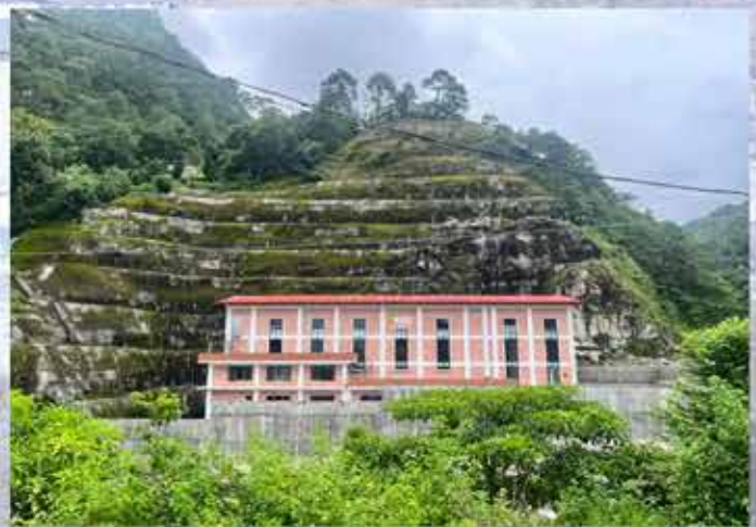
Khimti II Powerhouse 48.8 MW
