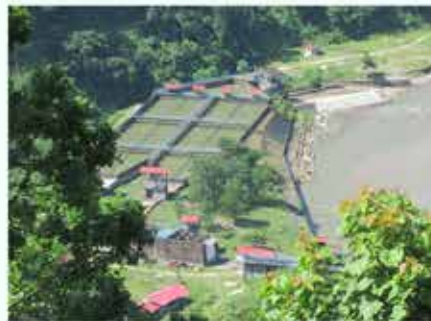
Mai Hydropower Plant (22 MW)
