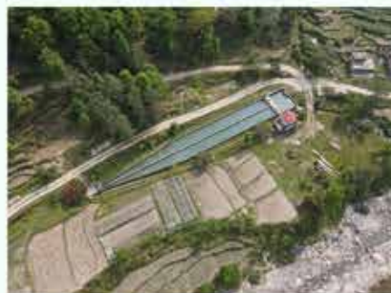
Sunkoshi Small Hydropower Plant (2.6 MW)
