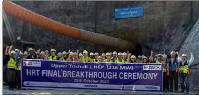
UT-1 Final Breakthrough of 9.5 km Headrace Tunnel
