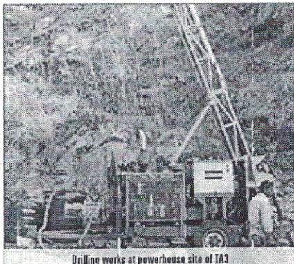
Drilling works at powerhouse site of TA3
