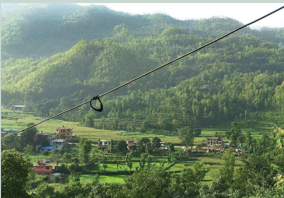
Photo of Power House Area of Middle Trishuli Ganga Hydropower Project (19.41 M.W.), Tupche, Nuwakot.
