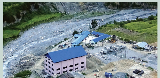
Power House and Switchyard Area of Thapa Khola Hydroelectric Project (13.6 M.W.), Tukucho, Mustang
